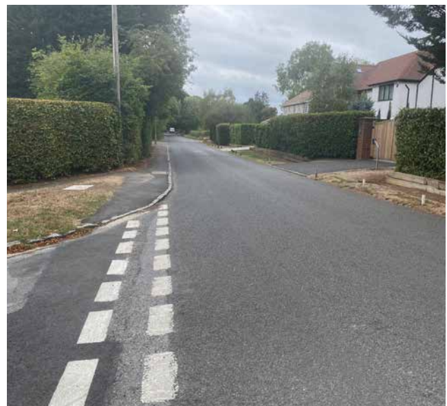
Figure 50: Local street displaying beech hedging as a popular boundary treatment in the local area, allowing it to keep its rural feel
