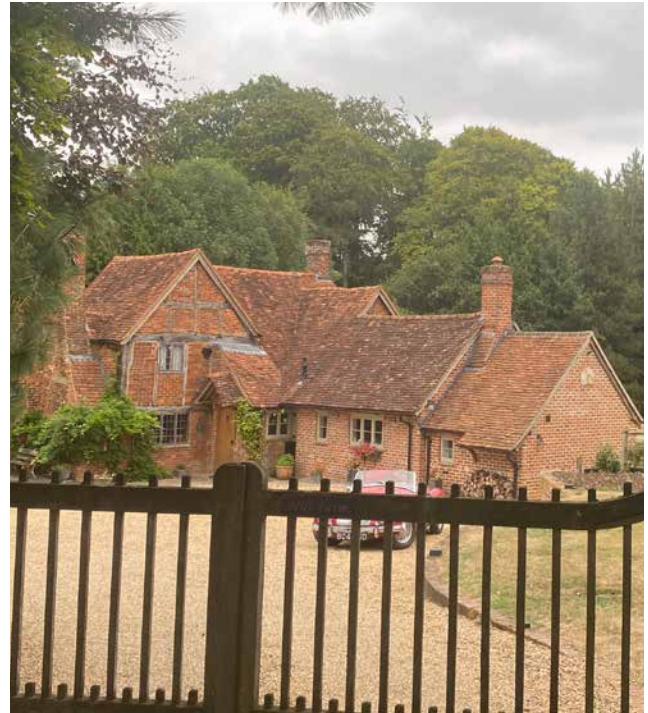
Figure 25: Listed building 'Hill Farm Cottage'
