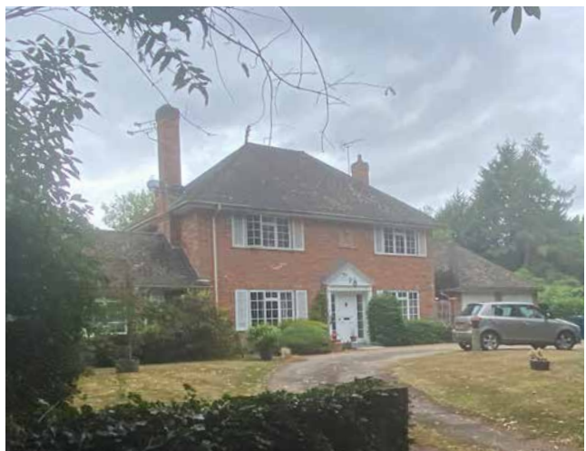
Figure 66: Generous front courtyard with on-plot parking within the parish. Knotty Green.
