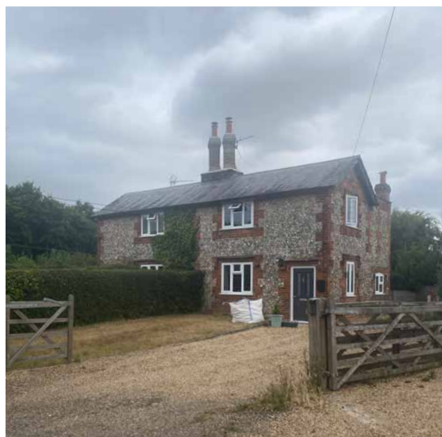
Figure 75: Detached flint house located in Penn Street.
